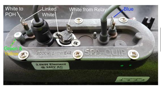
Incoloy Heater Element pre Nov 2015 wiring connections
