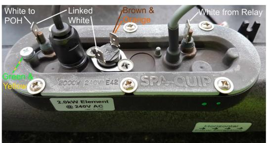
Incoloy Heater Element post Nov 2015 wiring connections
