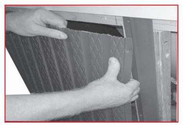
Starting at the left flange install the first panel as shown using three of the color matched screws. Use gloves to prevent cuts if panel edges are sharp.
