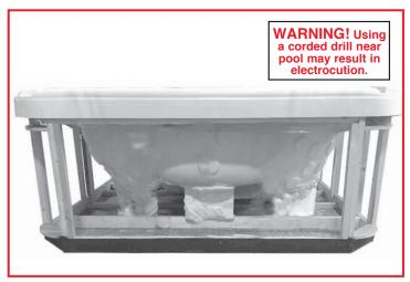
Deactivate the power to the spa. Remove the old skirting and measure the height. The new skirting will be installed the same way or butting up to the shell.
