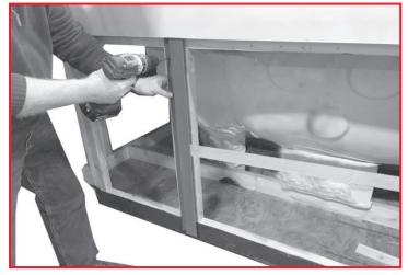
Using three screws in each flange, install both flanges onto each of the 2x4's used to frame out the service opening.
