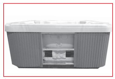
Continue installing the panels making sure to overlap at each end. The last panel will have to be cut in length to butt up to the flange edge.
