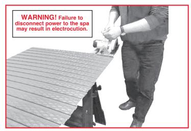
Using a circular saw with a fine tooth blade, cut all 5 panels and both flanges to this height. If using a corded saw, make all cuts a safe distance from the spa.
