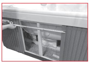
Measure from the outside of each flange and subtract 1" from that measurement. Cut a panel to length using this measurement.
