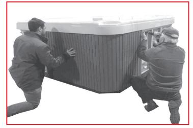
With a helper continue wrapping panel around spa keeping enough tension on panel to eliminate any buckling. Fasten panel into bracing using three of the provided screws in the top, middle, and bottom of the panel.
